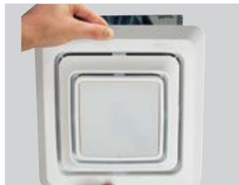
Attach new fan cover
